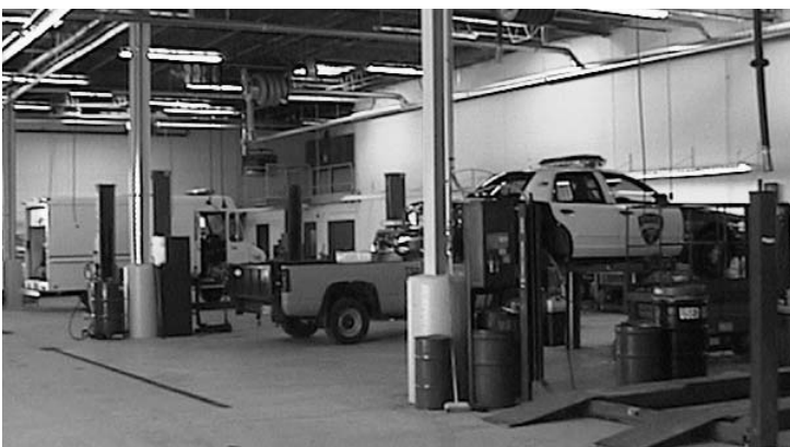
Part of the renovation of the new Public Works facility included the construction of a state-of-the-art mechanic's bay.
