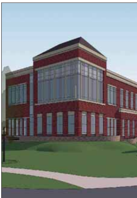
Northeast view of the new municipal building, respectively.
